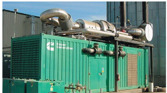
This cogeneration unit produces 1,250 kW of electricity, 2,200 pounds of steam and 30 gal/min of hot water, while besting local air-quality standards at a California animal feed processor.
