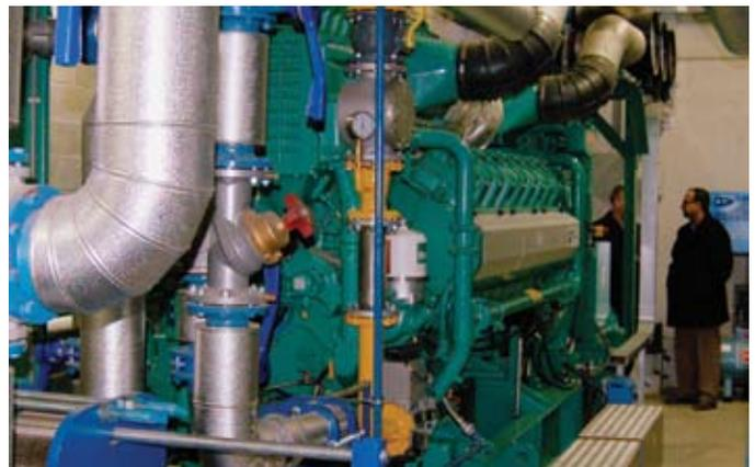
A 1.5 MW lean-burn gas generator set provides heat and power as well as CO<sub>2</sub> to accelerate the growth of tomatoes at a large greenhouse in Belgium.
